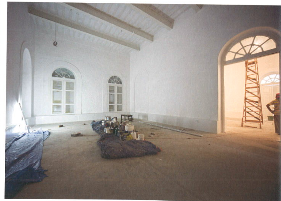
The Museum—renovation in progress
