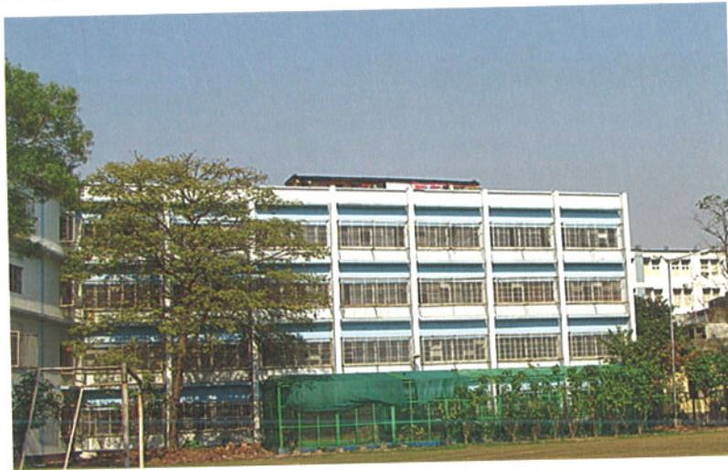
Netaji Subhas Building before renovation
