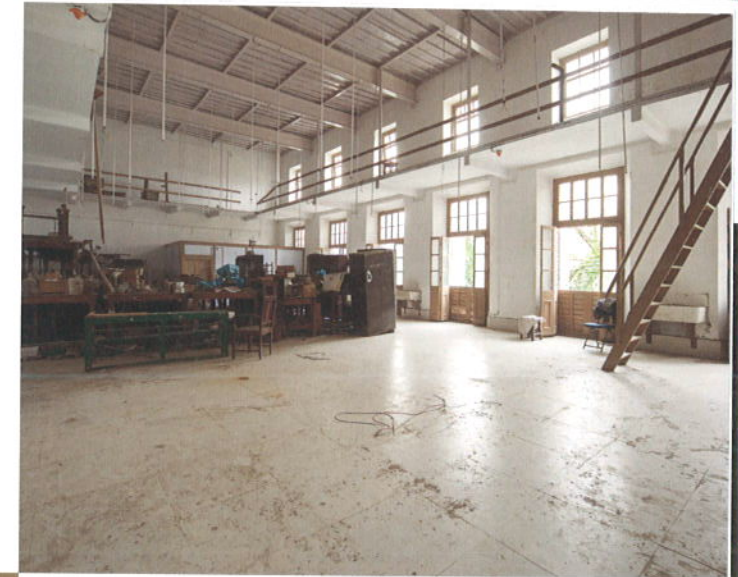
Renovation in progress
