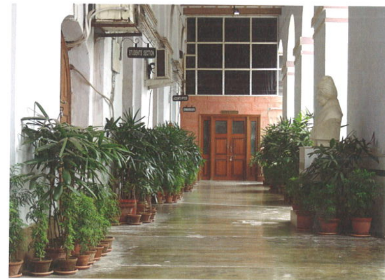
First floor corridor before renovation
