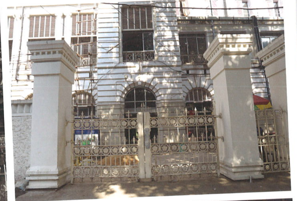
Heritage gate reinstalled at Baker Laboratories
